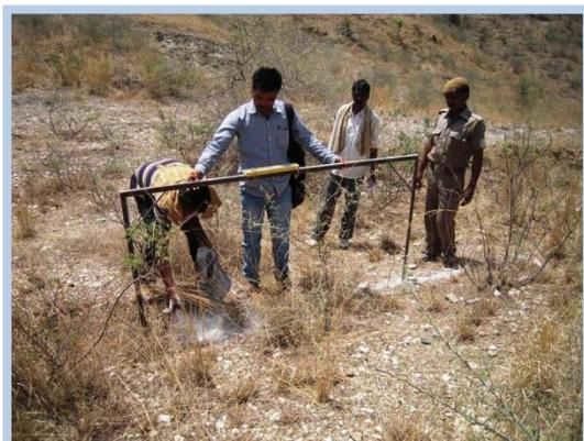
Fig. Marking contour line
